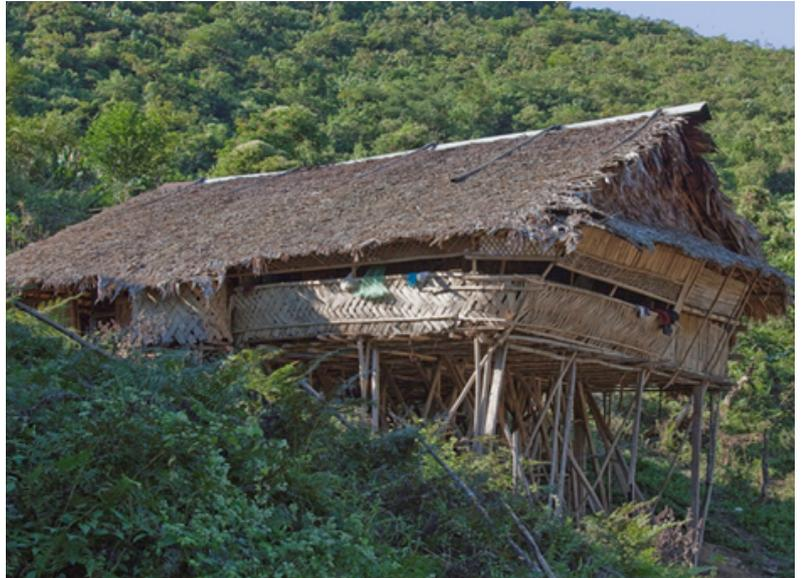
Using star palm leaves in roofing showcases an ingenious response to the region's climatic conditions. Thatch roofs, fashioned from these leaves, offer effective insulation against extreme temperatures while also maintaining an aesthetic charm.
