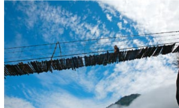
Cane bridges are commonplace in this part of the state
